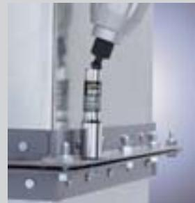
Tightening of duct coupling
