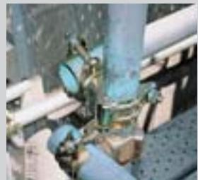
Tightening of step clamp
