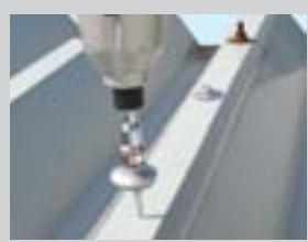
A ring nut setter is the best choice for securely fastening drill screws or flanged hexagon head screws with in high places as when anchoring angled plates in the middle.
