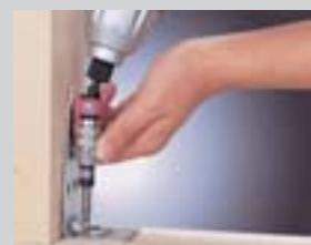
Installing tension and angle brackets
